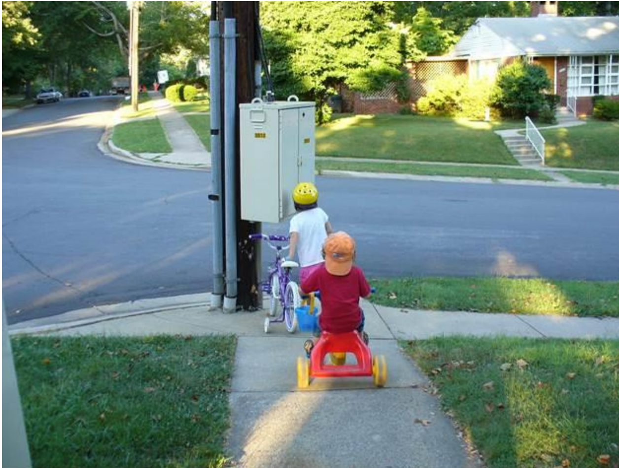
Pole – mounted version – Verizon FiOS cabinet
